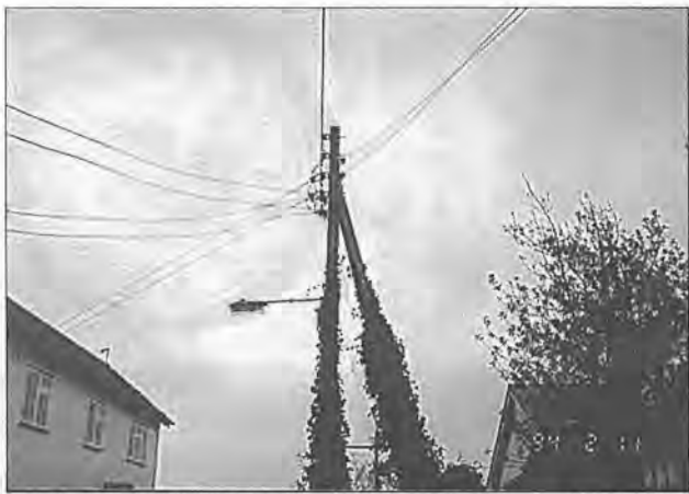
Some of North Wirral's overhead lines which have now been undergrounded.
